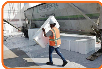
Construction improvements in progress
